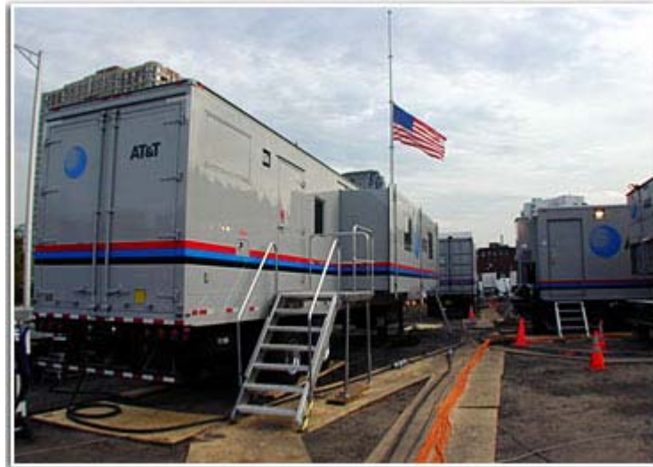
Figure 2.3.4.2-2: AT&T's Response to World Trade Center Disaster. AT&T's recovery equipment restored service within forty-eight hours after the loss of our central office in the World Trade Center.
